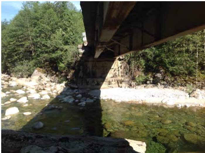
Left Bank Abutment when facing downstream
