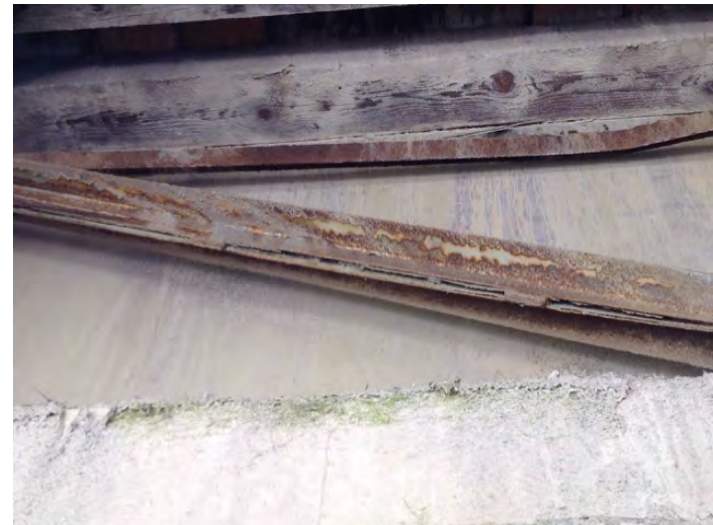
right abutment bracing
