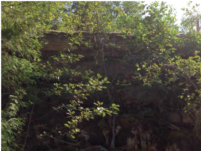
upstream left wing wall
