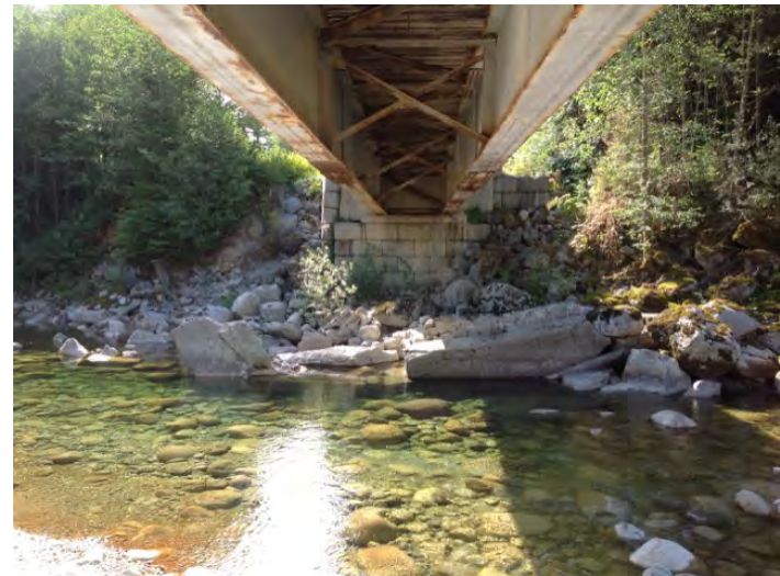
Right Bank Abutment when facing downstream
