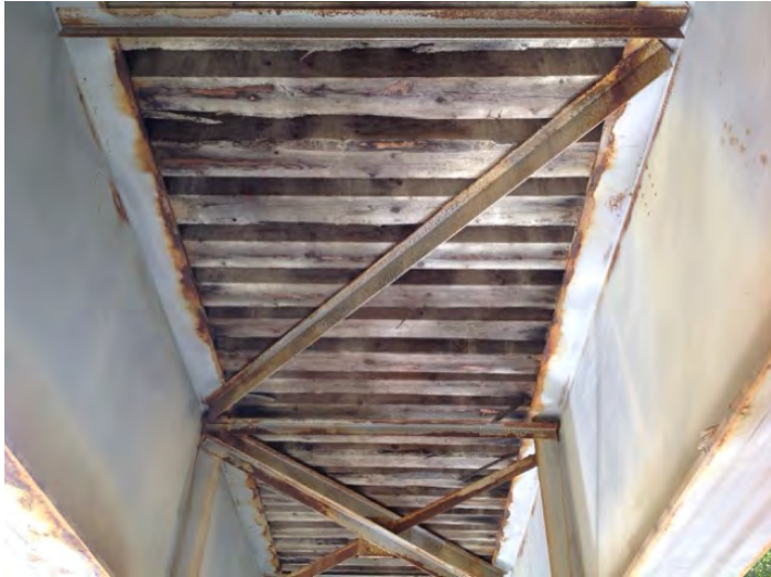
tie condition from underneath
