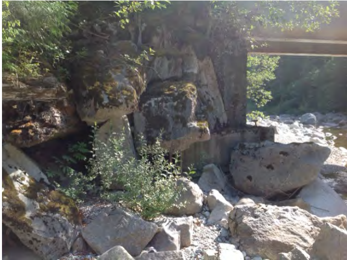
upstream left abutment
