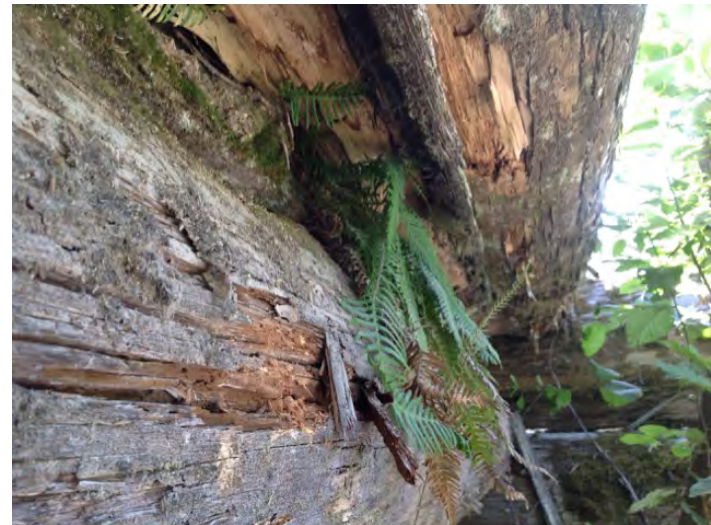
left upstream wing wall log condition - typical
